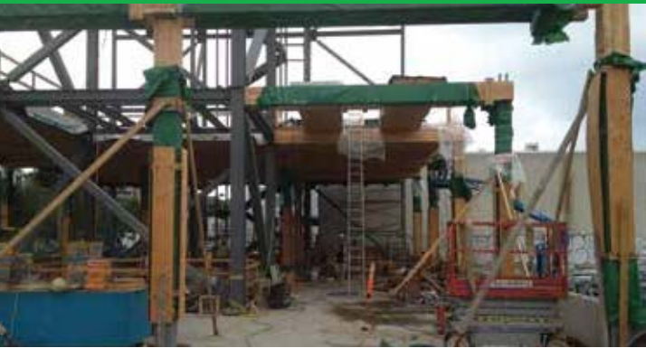
Erection of the post and beam structure Photo: Proscenium Architecture
