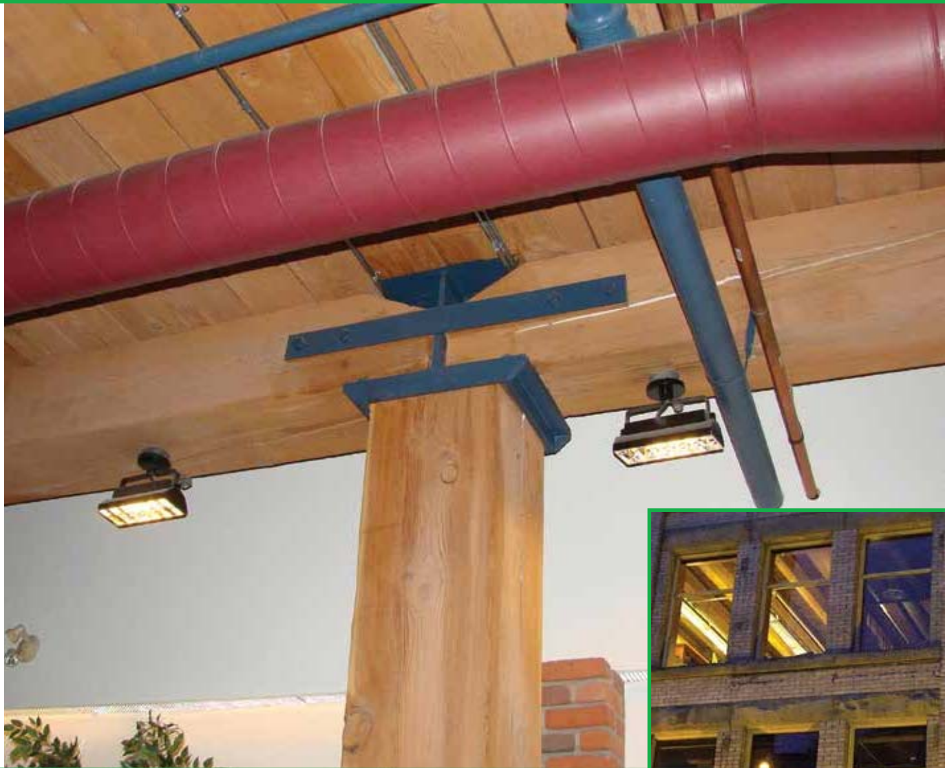
The Leckie Building (R) and Vancouver Building (inset). These impressive massive wood structures were built before the turn of the century in Gastown, Vancouver. The glulam beams in the Leckie Building (R) are supported off the glulam columns using a steel saddle detail. Photo: Courtesy, Wood WORKS! BC
