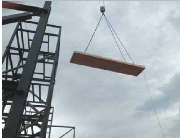
Floor panels were lifted into place by crane Courtesy: Proscenium Architecture
