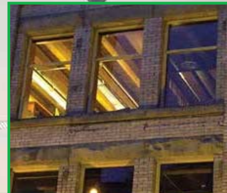
The Leckie Building (R) and Vancouver Building (inset). These impressive massive wood structures were built before the turn of the century in Gastown, Vancouver. The glulam beams in the Leckie Building (R) are supported off the glulam columns using a steel saddle detail. Photo: Courtesy, Wood WORKS! BC
