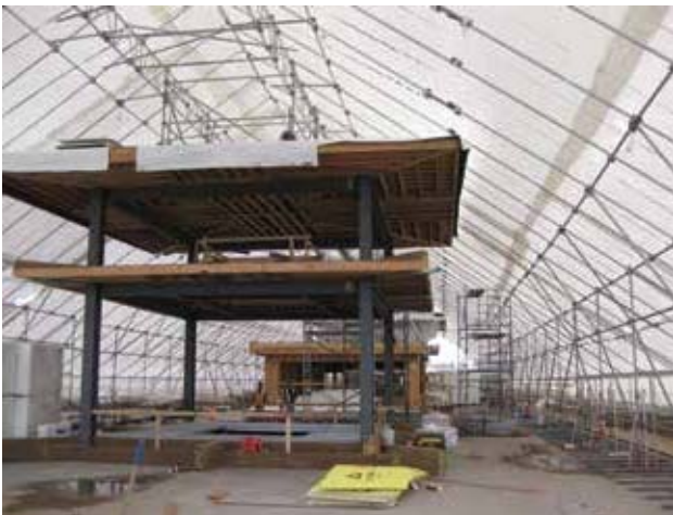
A tent was erected to protect the wood structure from inclement weather during erection and prior to closing in Courtesy: Proscenium Architecture
