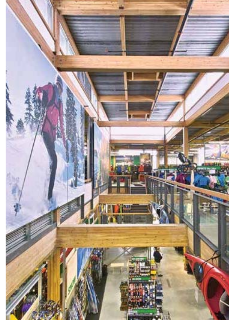
Above: MEC, Burlington, ON This store was designed with a completely demountable heavy timber structure Courtesy: MEC
