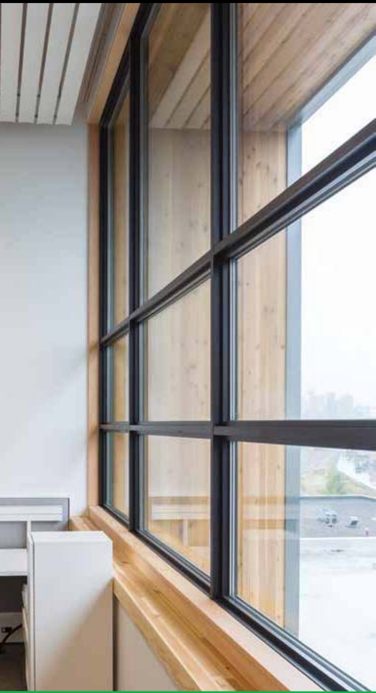
Detail of window Photo: Ed White Photographics
