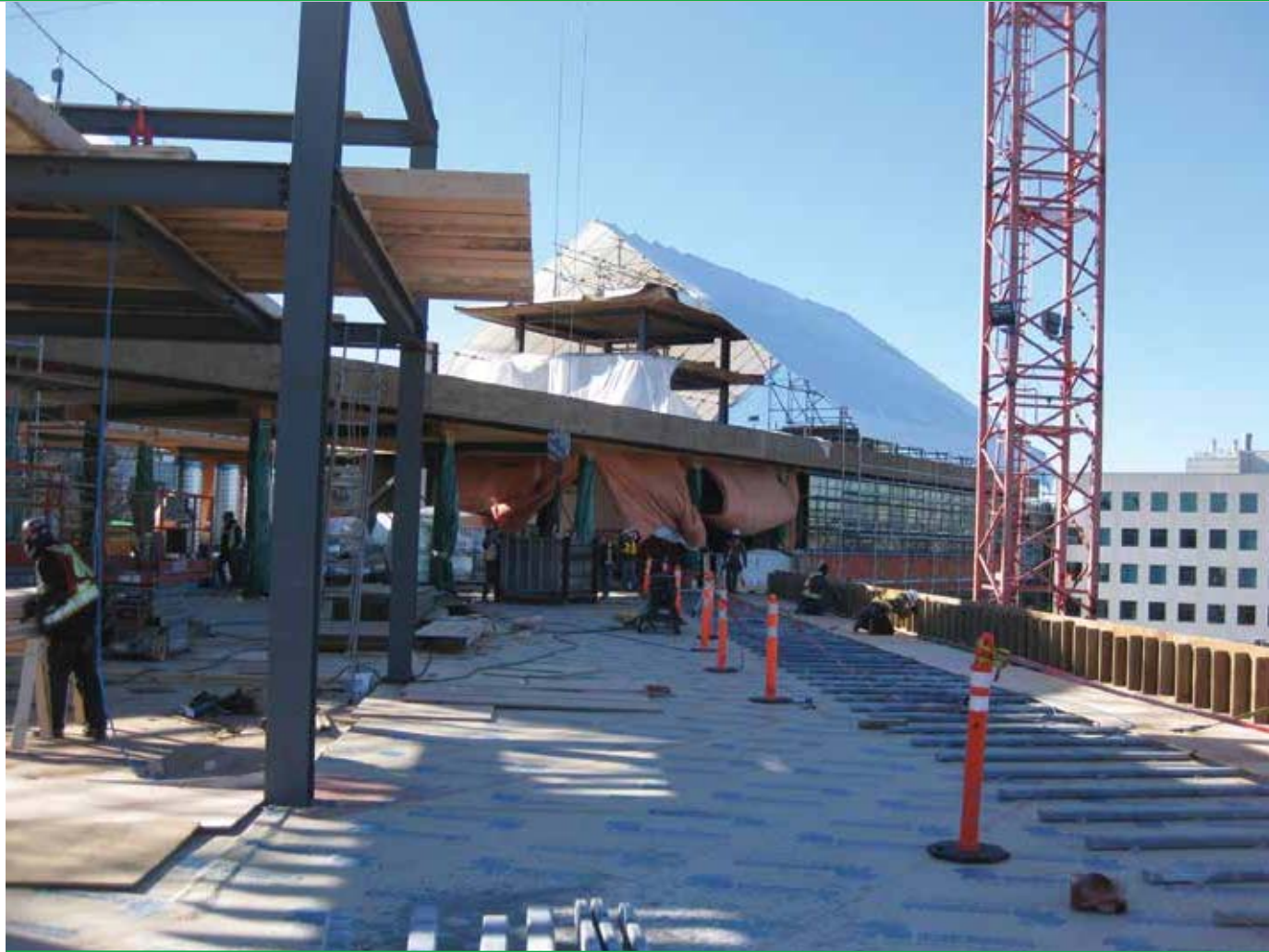
A tent was erected to protect the wood structure from inclement weather during erection and prior to closing in Courtesy: Proscenium Architecture
