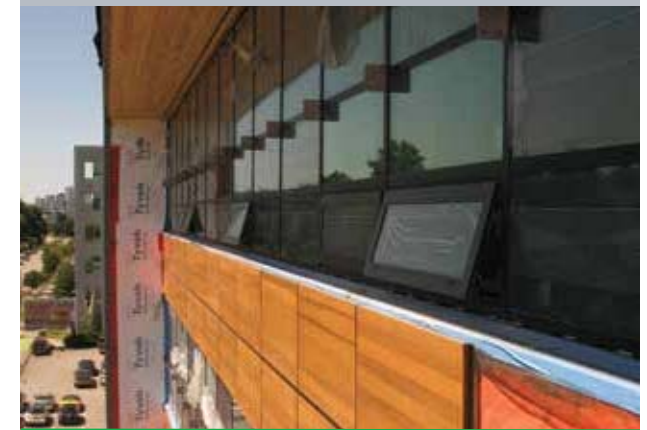
Detail of cladding installation Courtesy: Jim Taggart
