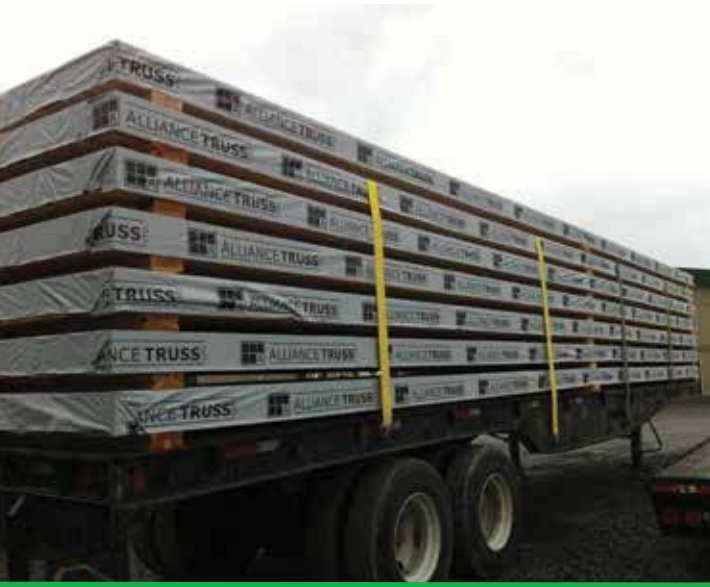
Prefabricated floor panels are delivered to site for installation Courtesy: Fast + Epp
