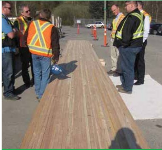
Factory prefabrication of nail-laminated floor panels Courtesy: Proscenium Architecture
